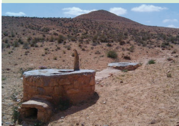
Water collected in a cistern: the water is used for household and livestock production. Photo: Ouessar M., Tunisia
