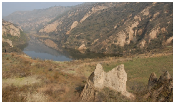
A check dam in the Loess Plateau of China provides and traps sediment until it is filled up. It is then used for crop production.
