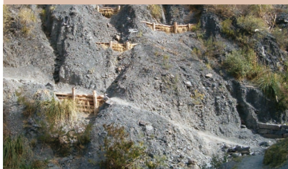
Catchment gully control in Bolivia with a variety of different SLM technologies. Photo: Georg Heim
